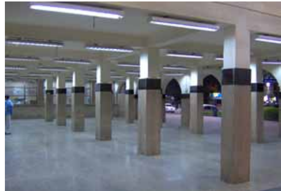
Secunderabad concourse T5 lighting
