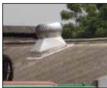
Roof Ventilators
