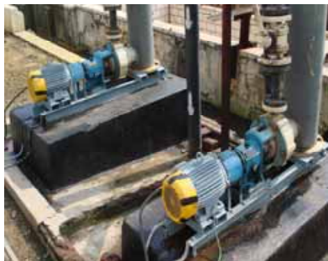
New High Efficiency PP Pumps For ETP Collection Tank With PP Self Priming Pot & 5 HP/2900 RPM, EFF1 Level Motor
