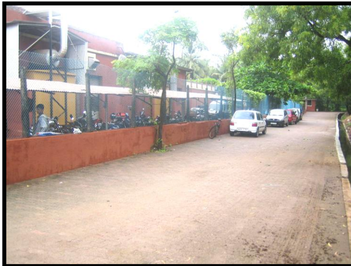
Used pavers utilized for construction of road
