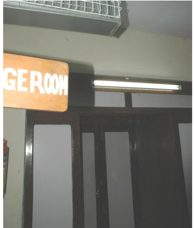
T-5 tube light 2x28W fitting
