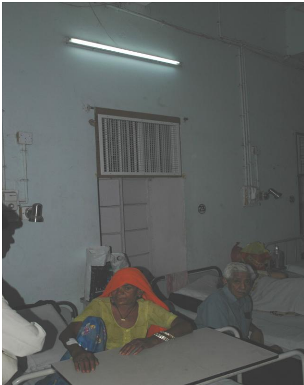
T-5 tube light 1x28W fitting
