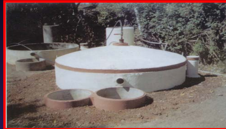
Biogas Plant For Canteen
