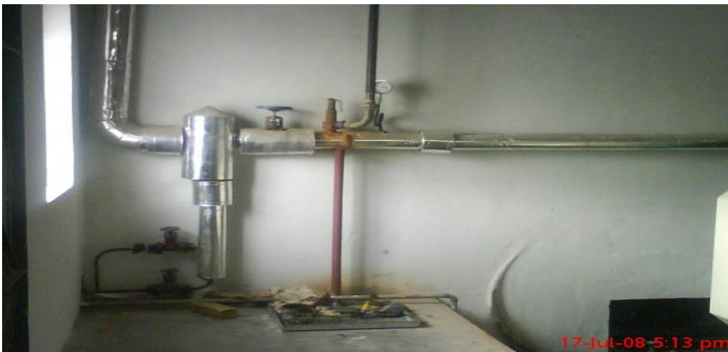
STEAM HEATING ARRANGEMENT
