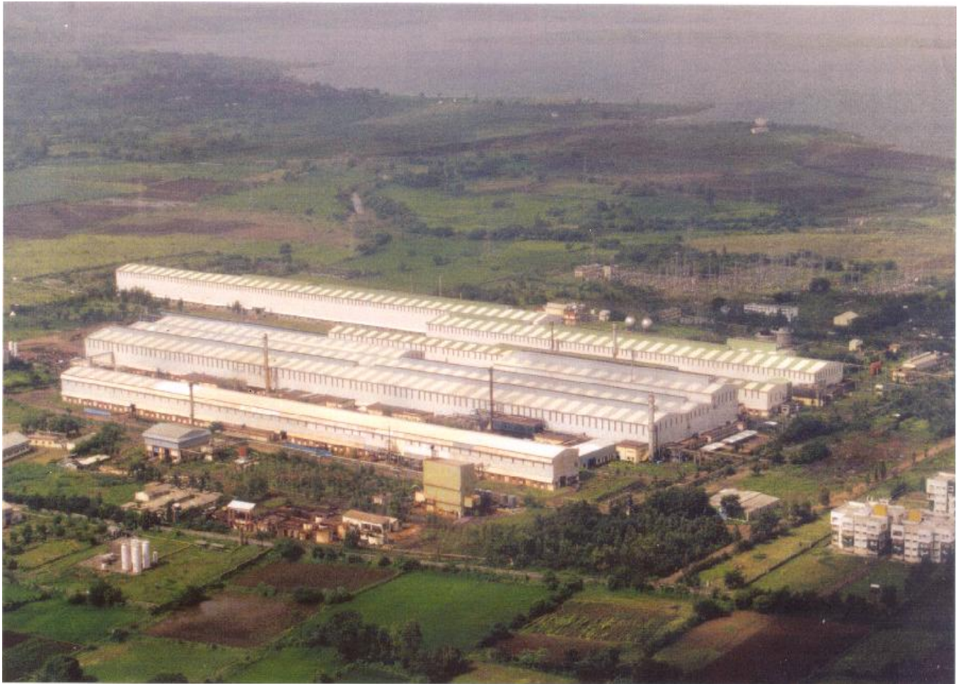
ThyssenKrupp Electrical Steel India Private Limited At Post - Gonde, Village - Wadivarhe, Tal - Igatpuri, Dist - Nashik, Maharashtra
