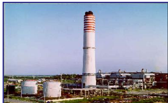
Captive Power Plant
