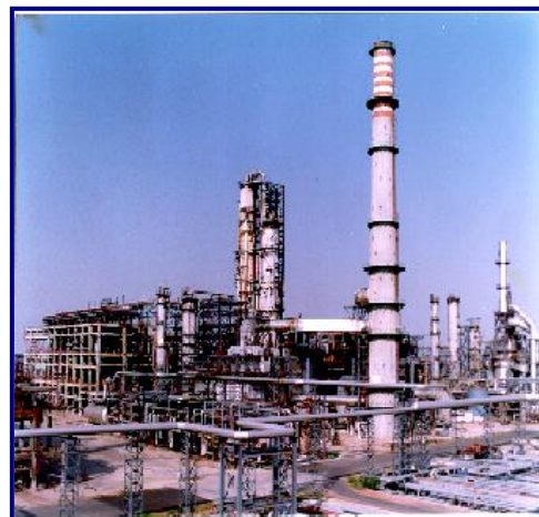
Crude Distillation Unit-1
