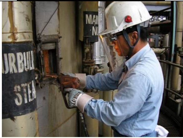
Chemical spraying in progress
