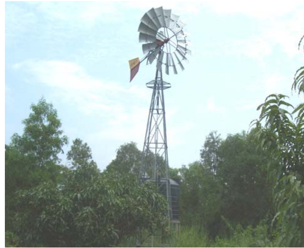
water Harvesting Project
