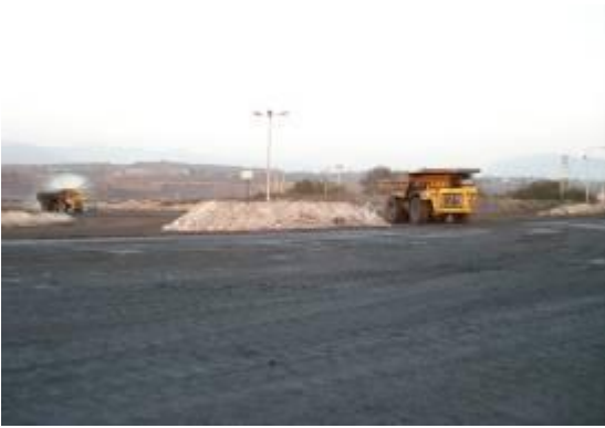
Safe and Wide Haul Road with Island
