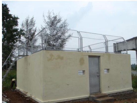
solid waste disposal yard
