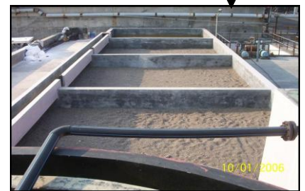
Top view of sludge drying beds
