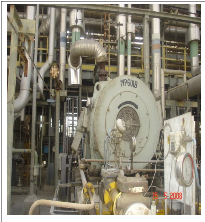
Removal of stage from Boiler feed pump of Ammonia plant
