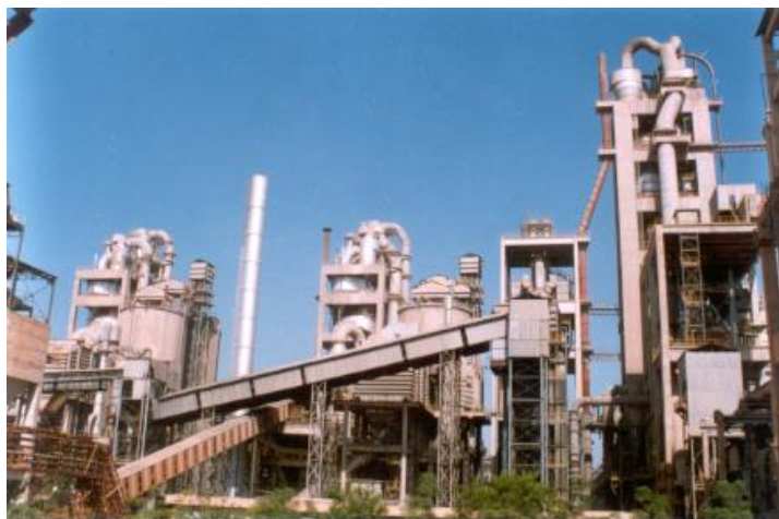
PLANT VIEW - VIKRAM CEMENT LINE-1 IS FIRST FROM LEFT
