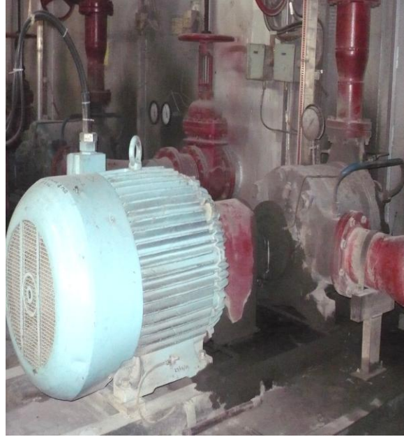
ROLL COOLENT FEED PUMP AC MOTOR
