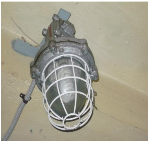
27 W CFL in place of 160 W mercury lamp
