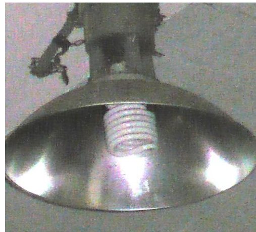
90 W CFL in place of 150W HPSV lamp
