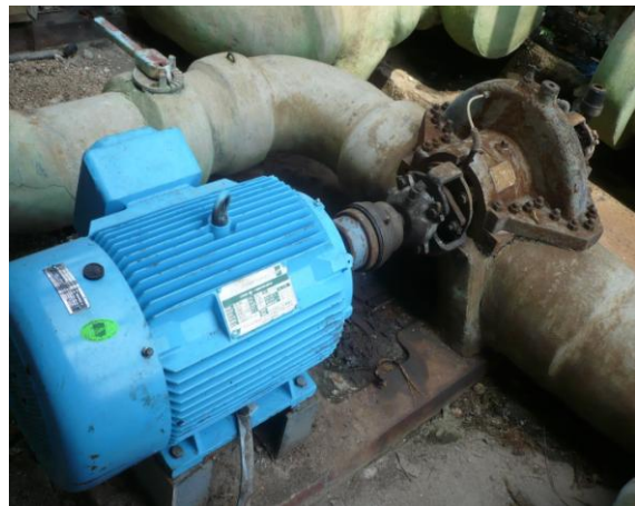
IN CASTER COLD WATER CIRCULATING PUMPS
