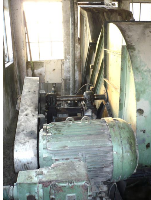
FUME EXHAUST SYSTEM : 75 KW AC MOTOR
