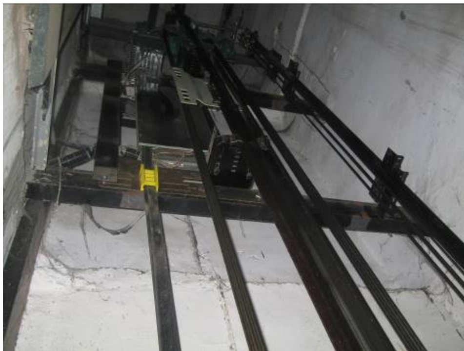
Replacement of old 11 KW electric motor with VVF 6 KW AC electric motor at New Delhi Railway station
