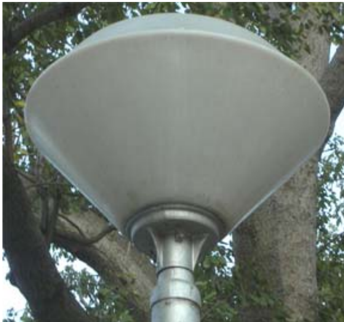
Old 70 Watts HPSV Compound Light Fitting
