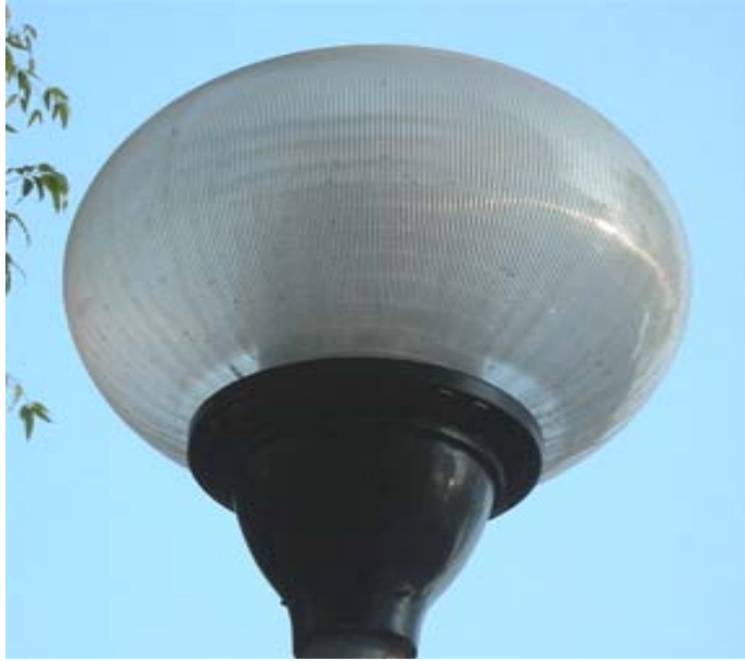
New 28 Watts CFL Compound light fitting
