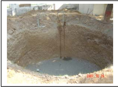
Rain Water Harvesting Pit (Work in progress)
