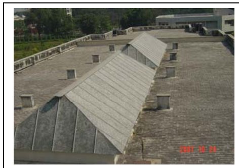
Roof With Transparent Fibre Sheet
