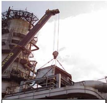
Removal of the old Module
