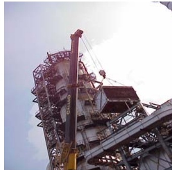
Installation of the new Module
