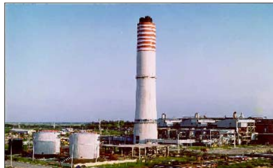
Captive Power Plant
