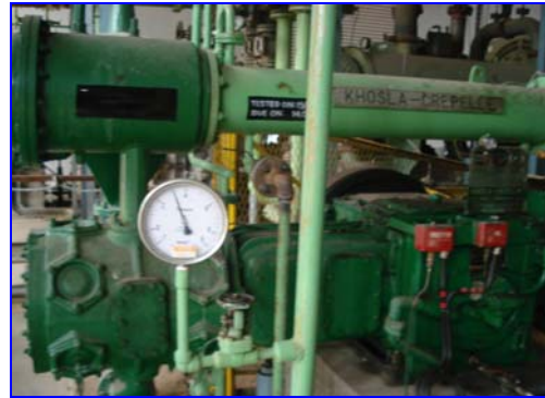
2 Nos. of LT reciprocating compressor of lower capacity 600NM 3 /Hr. were installed. Other available compressor 2100 NM 3 /Hr. Capacity made operational.
