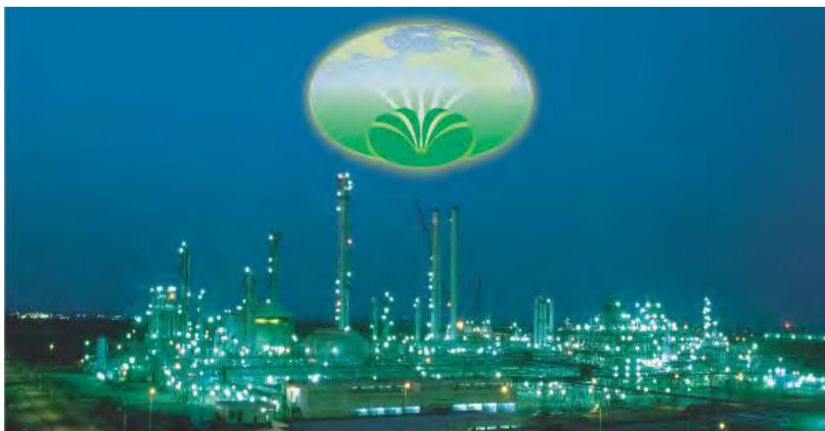
(Photograph of RIL, Vadodara Mfg. Div. where detailed audit of steam traps of whole site was done)
