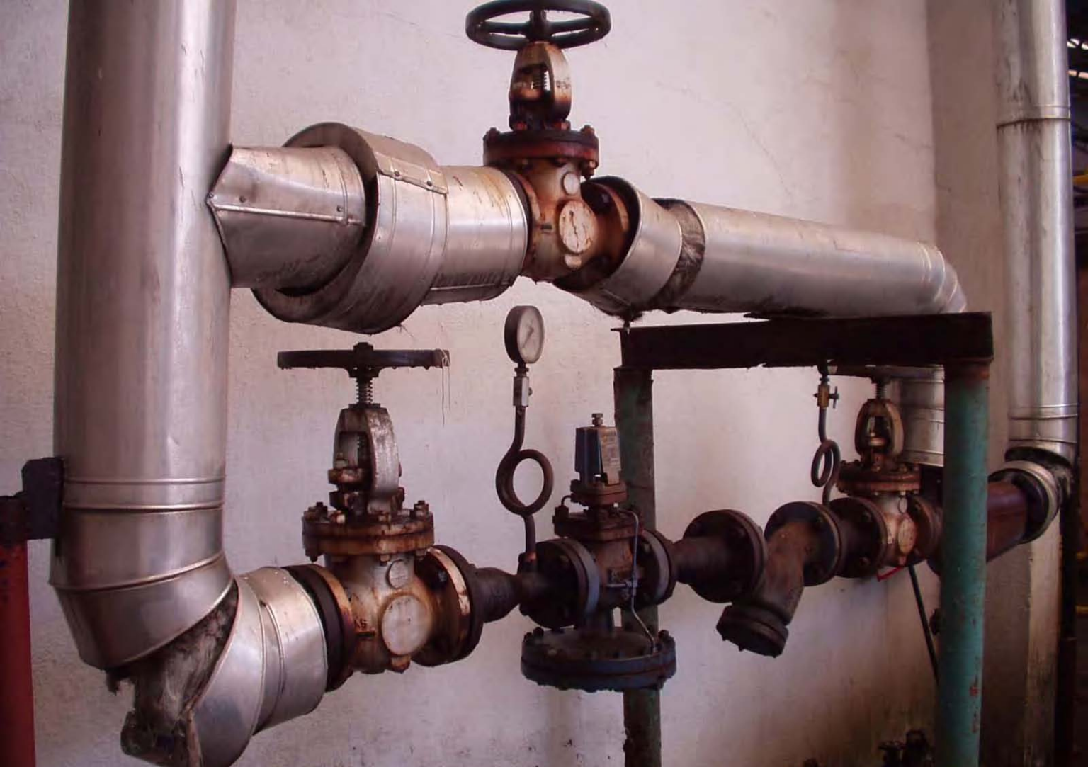
PRV station -Viscosity Index Improver Plant
