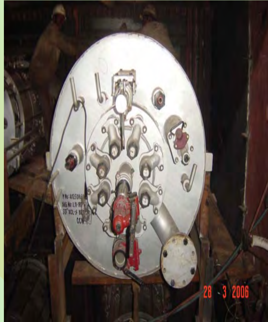
View of Dual Firing Burners in Boiler # 4
