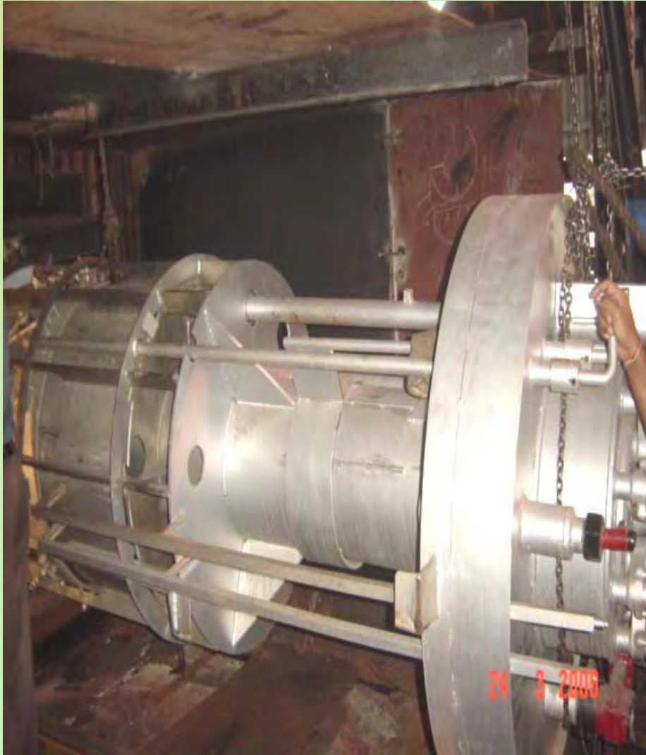
View of Dual Firing Burners in Boiler # 4
