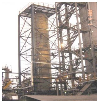
S-50 Synthesis Converter with Waste Heat Boiler
