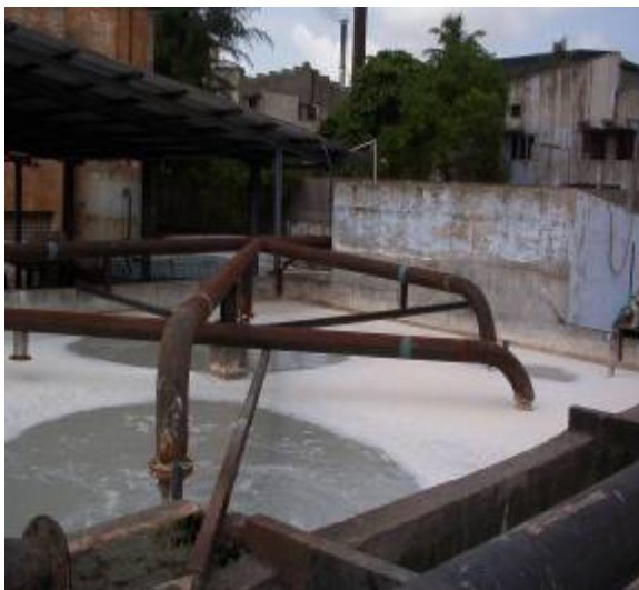
OLD ETP PLANT
