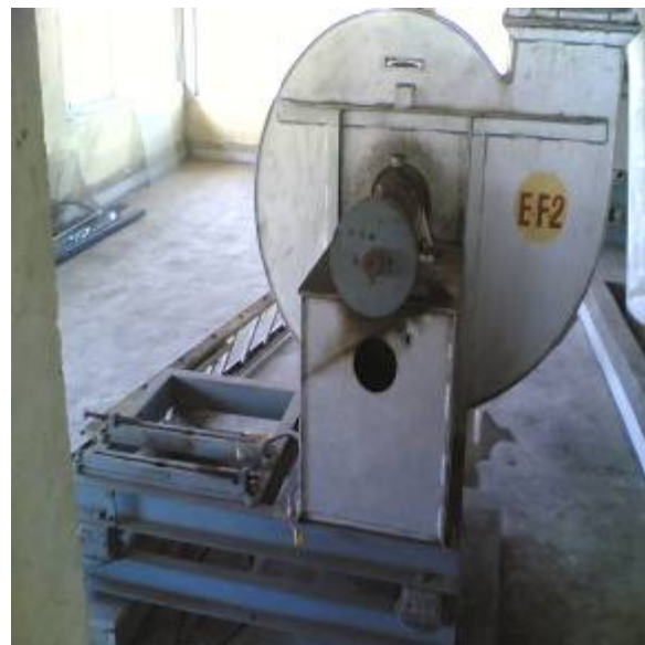
Exhaust fan after removal
