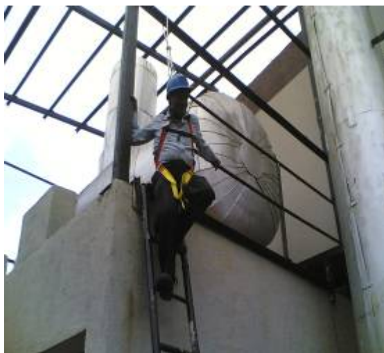
SAFETY BELTS DURING WORK AT HEIGHT
