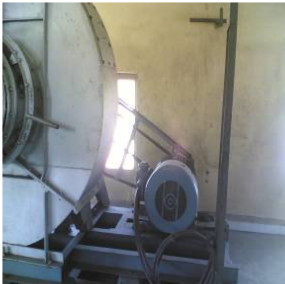
Exhaust fan before removal
