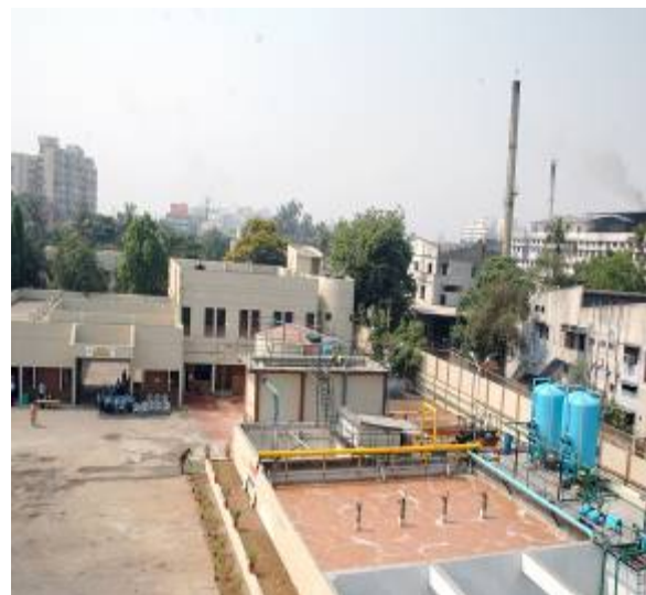
NEW ETP PLANT
