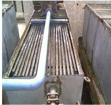
DESCALED COILS
