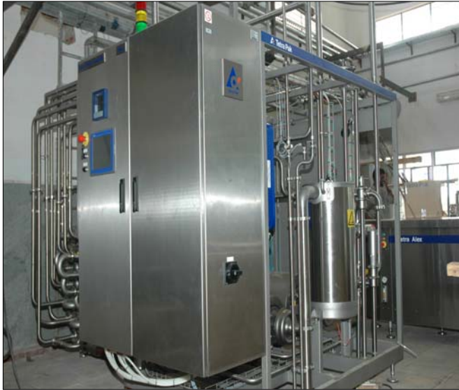
UHT Processing Plant
