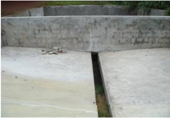
New Sand filtration beds under construction.
