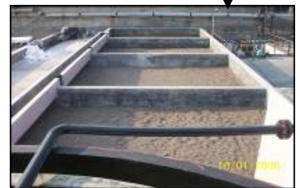
Top view of sludge drying beds
