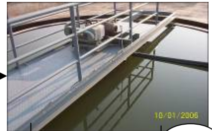
Top view of clarifier
