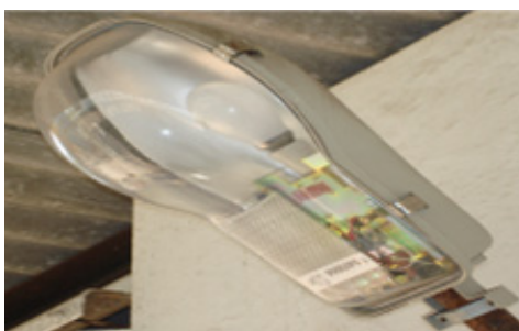
New 70 W Energy efficient Sodium Vapor Lamps
