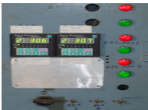
Delta-T Controller For Cooling Tower Fans
