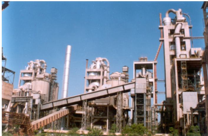
PLANT VIEW - VIKRAM CEMENT LINE-III IS FIRST FROM RIGHT
