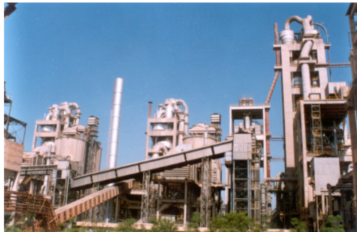
PLANT VIEW - VIKRAM CEMENT LINE-II AT CENTER
