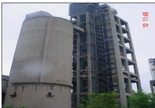
RABH ,MAIN CHIMNEY & PRE-HEATER
