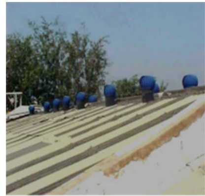
Use of natural ventilation
