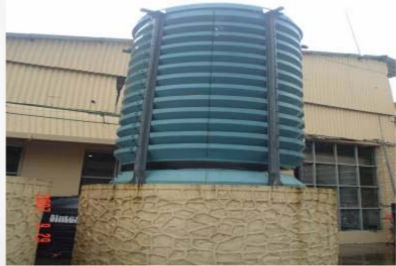
Fanless natural draft cooling tower Energy cost- Nil
