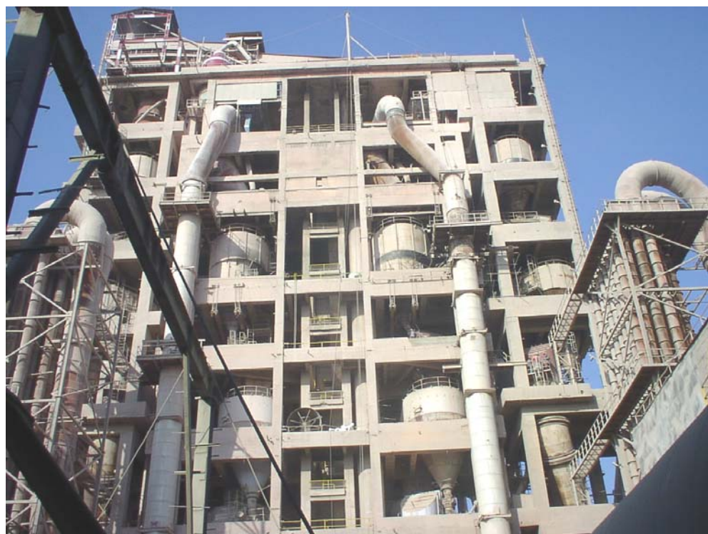
Preheater Tower of Kilns
