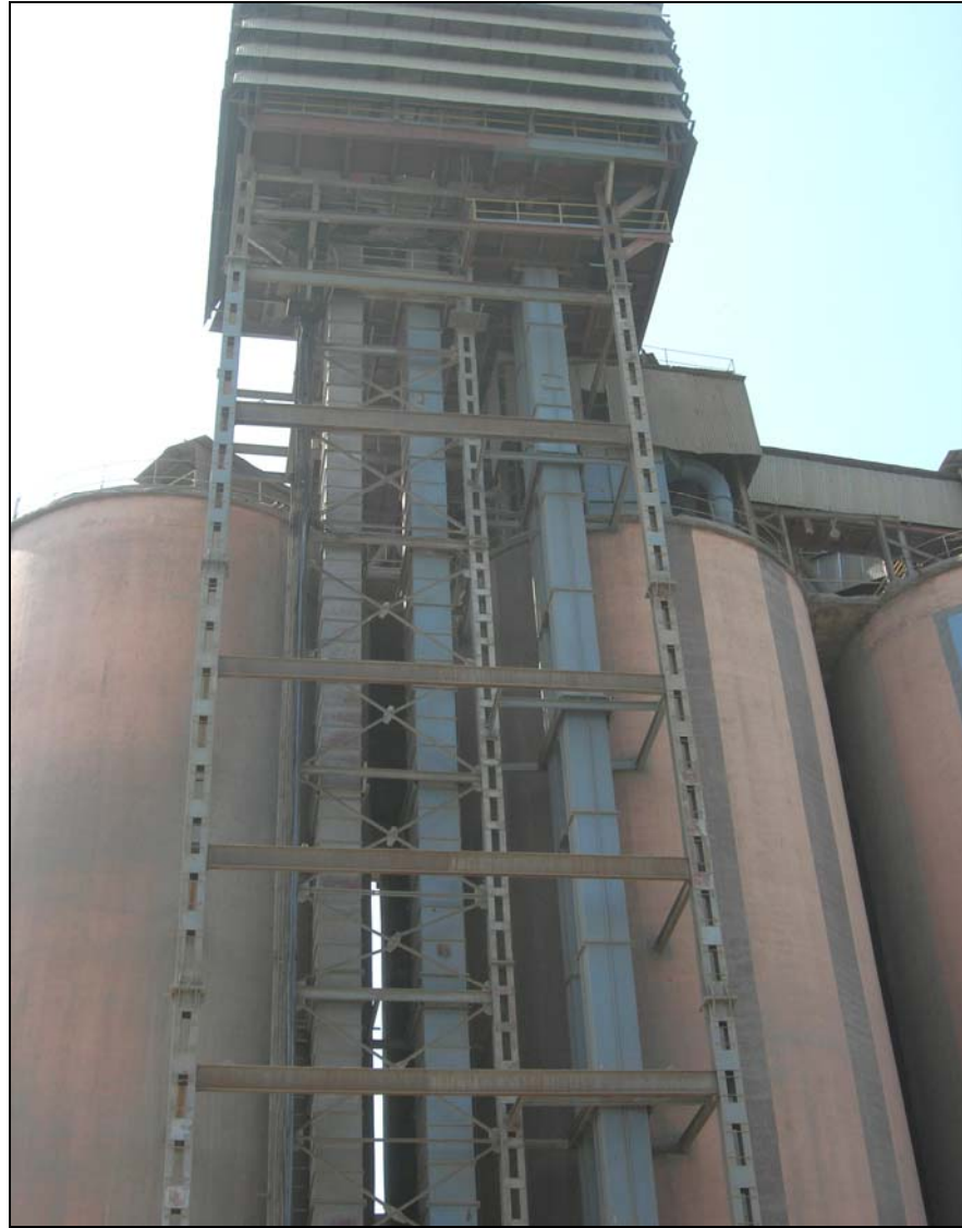
Mechanical Transport System
