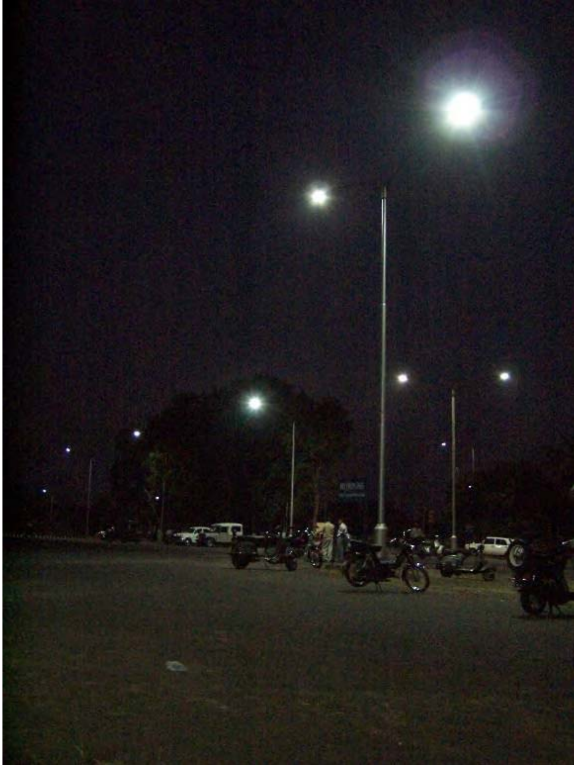
In the Sachivalaya Complex campus there were 200 Nos. of Street Light fittings installed on poles for street light (Compound Lighting)
