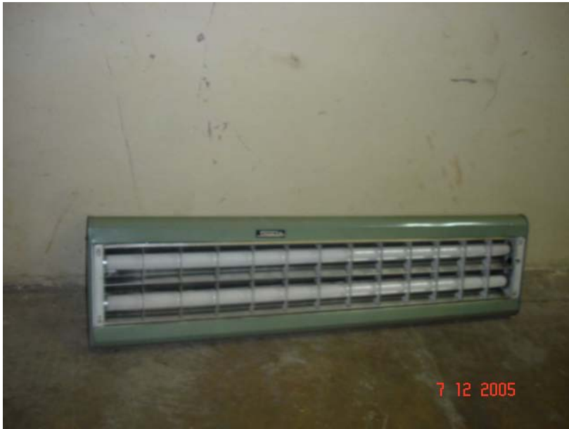
Old 2x40 w fittings replaced
