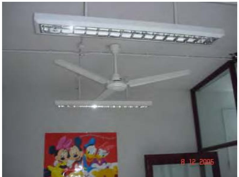
Energy saver T-5 (28W) fitting installed
