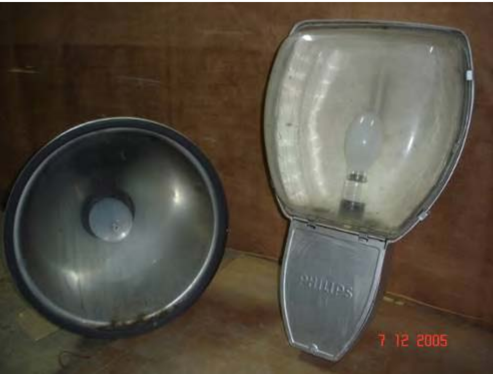
400 W halogen / HPSV lamps replaced
