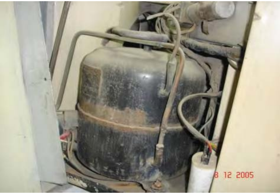
Old faulty reciprocating Compressors in Window AC units replaced
