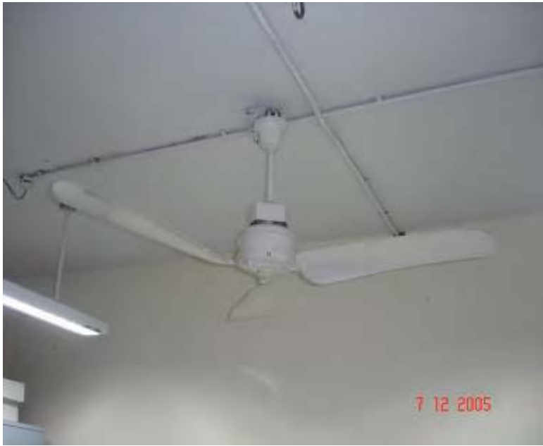
Old ceiling fans consuming more energy replaced
