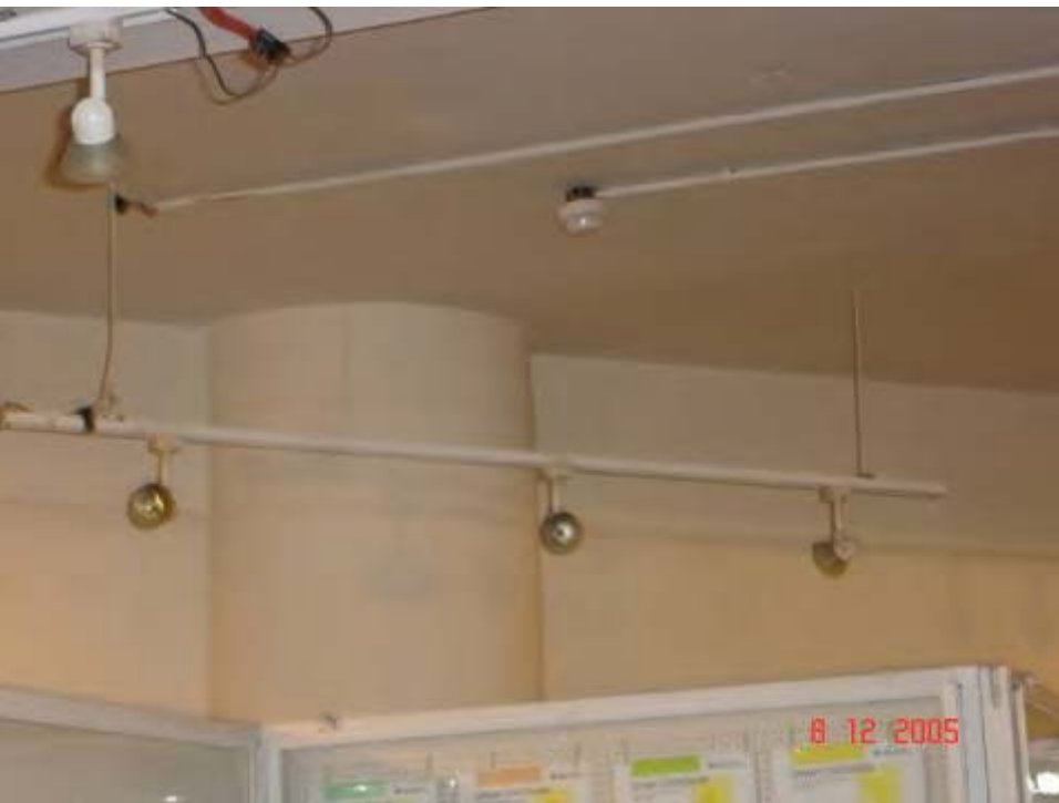
Halogen dichroic 50 W lamps in Philatelic Museum replaced
