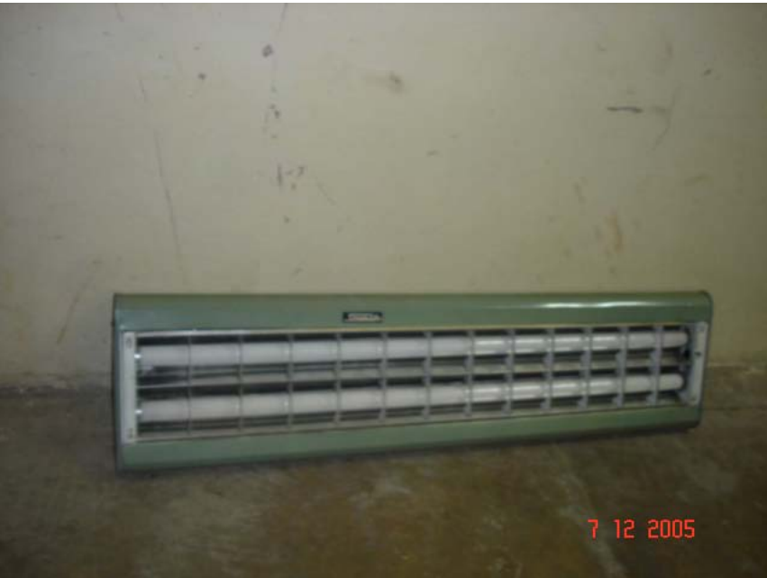
Old 2x40 w fittings replaced
