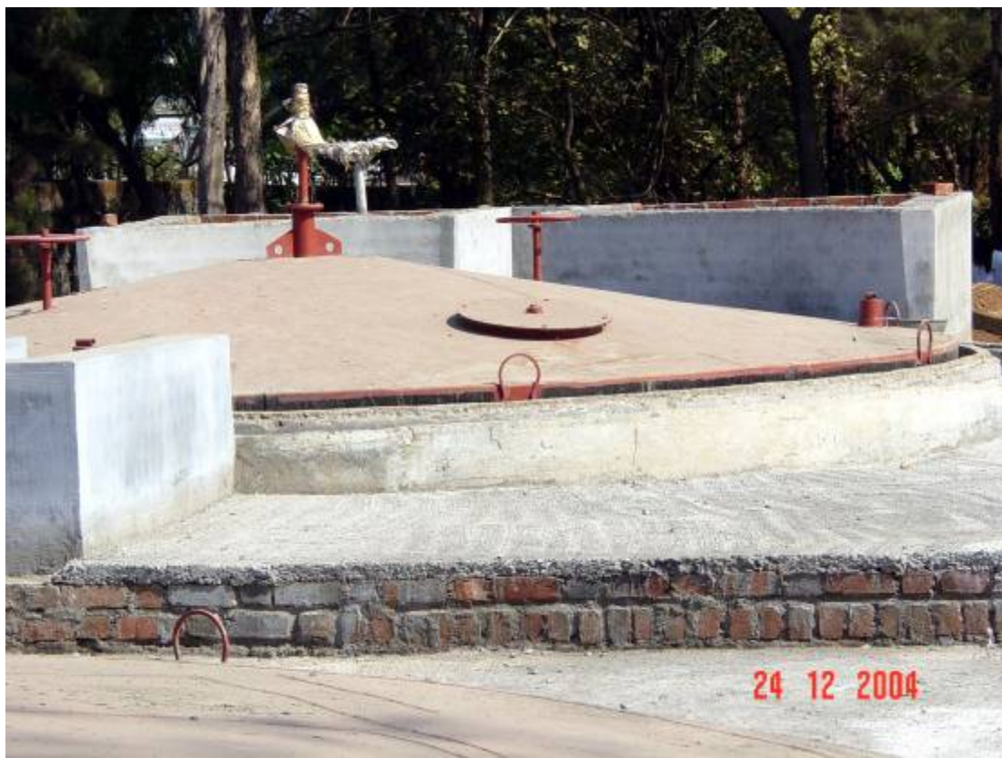
METHANE GAS PLANT FROM BIODEGRADABLE WASTE
