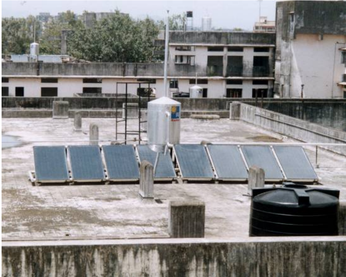
SOLAR WATER HEATING SYSTEM (TOTAL 19050 LPD)
