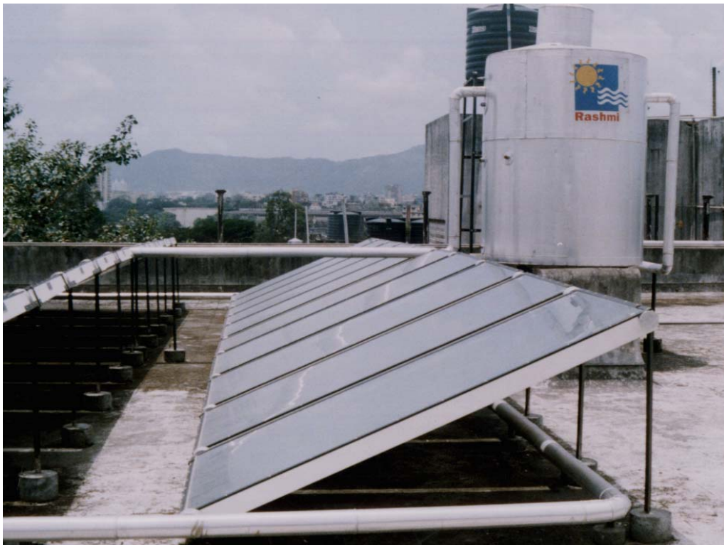
SOLAR WATER HEATING SYSTEM (TOTAL 19050 LPD)
