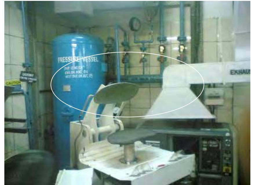
The highlighted place determines the place of installation of receiver and PRV in the outlet line of the compressor
