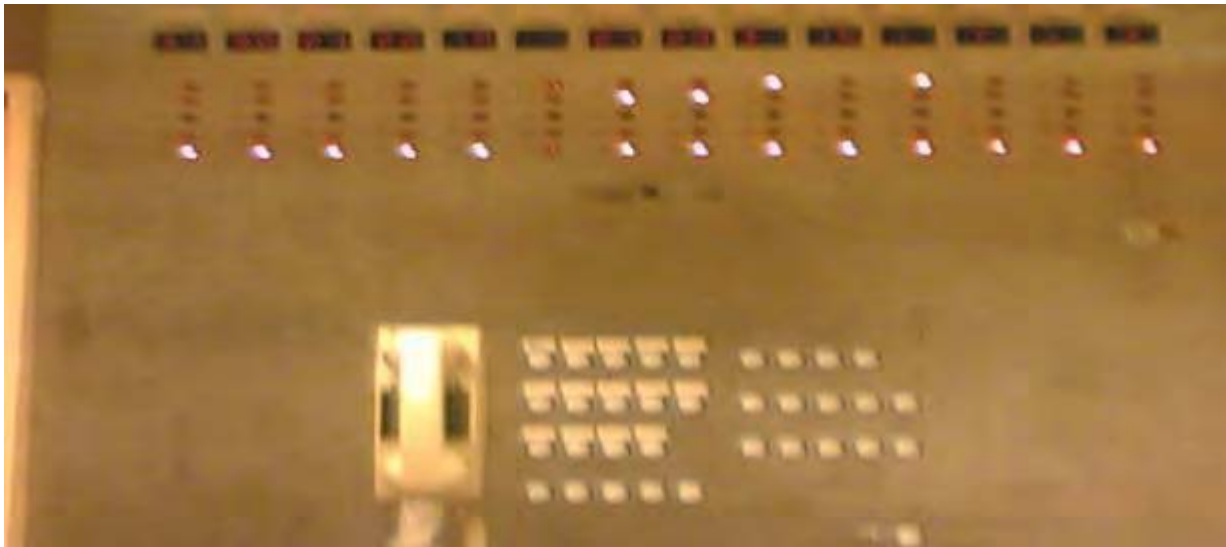
Above shown is the manual rescue call receiving centre of the elevators
