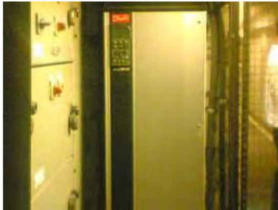
Installed VFD
