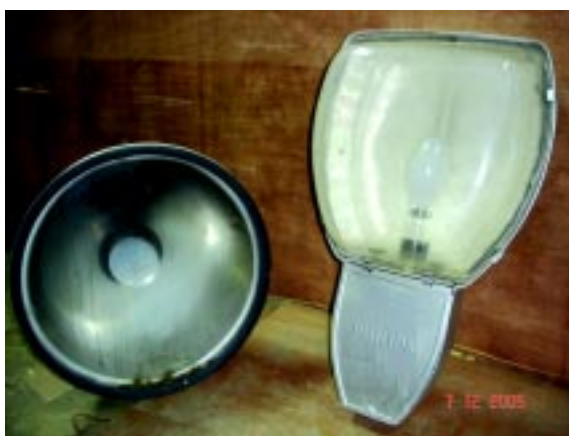
400 W halogen / HPSV lamps replaced
