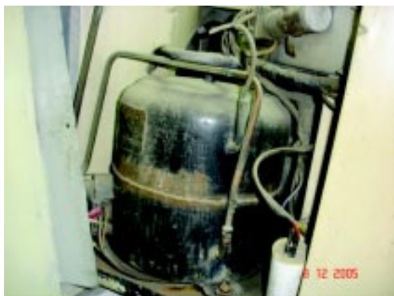
Old faulty reciprocating Compressors in Window AC units replaced
