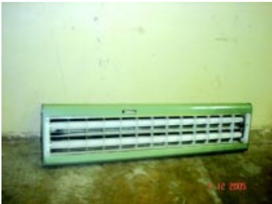
Old 2x40 w fittings replaced
