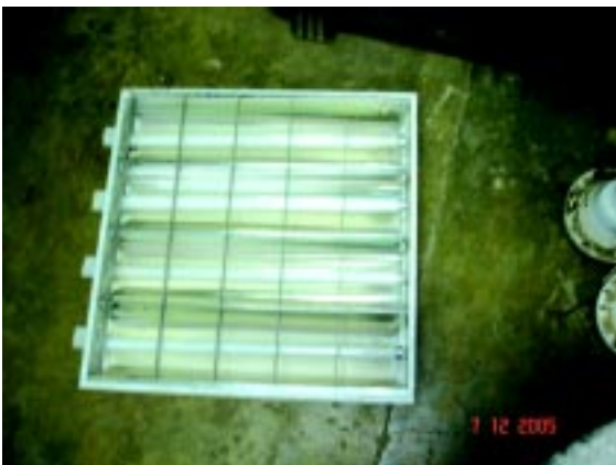
4x20 w fittings Replaced
