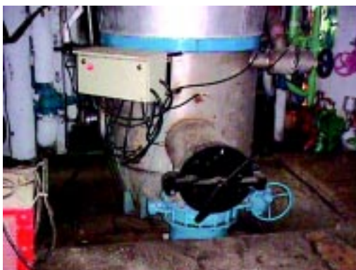
SPRAY EJECTOR CONDENSER
