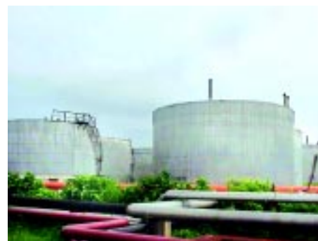
700 Tank Farm – After Insulation
