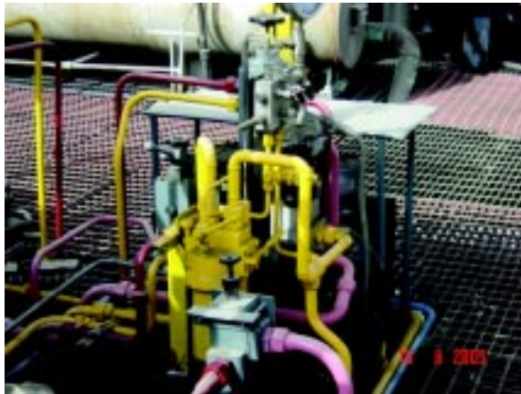
View of Governing oil Console and I/H Converter of Electronic Governor.
