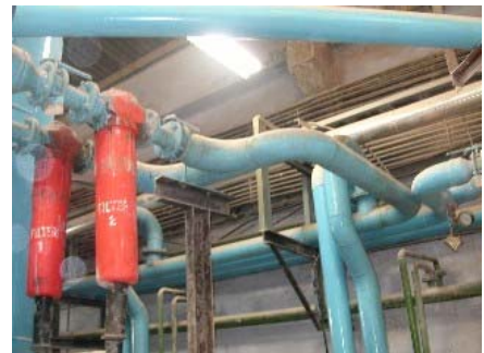
COMPRESSED AIR DISTRIBUTION
