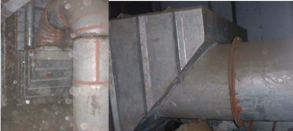
BENDS IN H.TOWERS MODIFICATION IN DUCTING OF H.TOWERS
