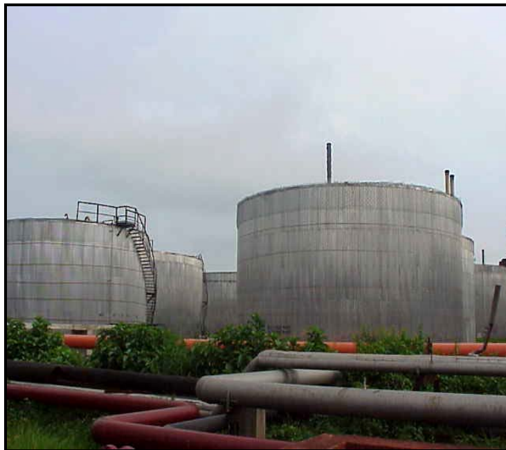
700 Tank Farm – After Insulation
